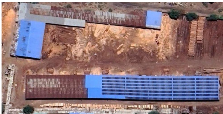
Kamal Timber – 250KW
